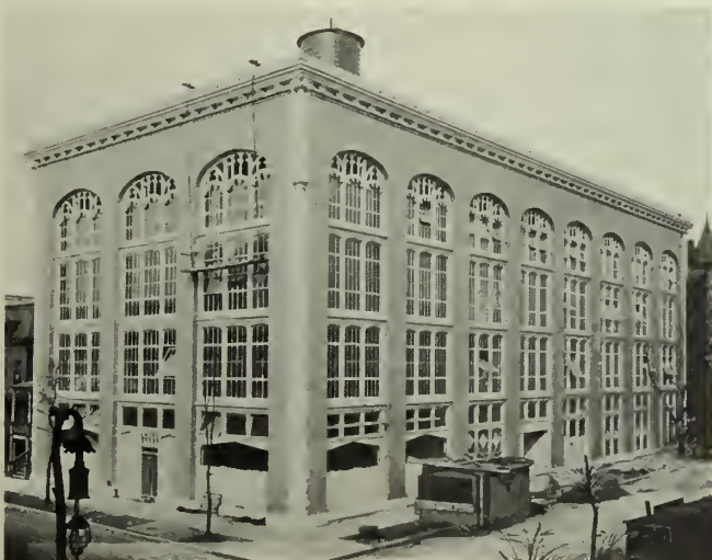
AUTOMOBILE SALES BUILDING, CHICAGO. Cream enameled terra cotta trimmings made by the Northwestern Terra Cotta Company. Holabird & Roche, Architects.
